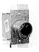
Throughout the following steps, make sure the control cable is kept accessible and protected from damage. It will be needed later to connect the control.
