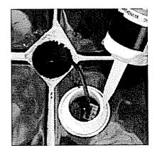
Clean the wall surface to ensure the silicone will adhere then place the control into the hole and tape in place until the silicone cures.
