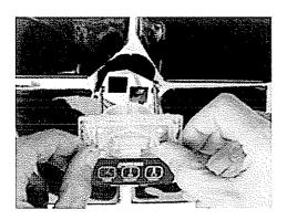
Tighten the bracket screws until the control is pulled snuggly against the wall. Do not over tighten – this may damage the control and cause vapor leaks!
